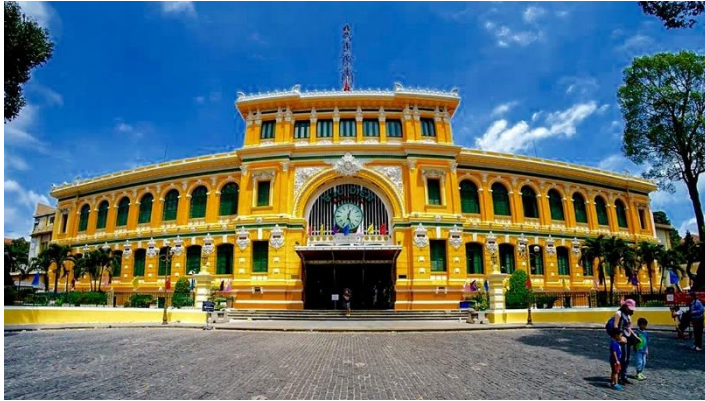
Picture from trungydang on Panoramio under Creative Commons License
